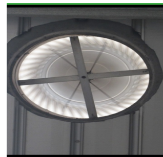
Installation of Turbo-Ventilators in Utility Shades & CPCP
