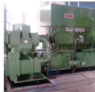
Advanced Turbo Compressor with inlet guide vanes, energy efficient control logic and 11kv Motor
