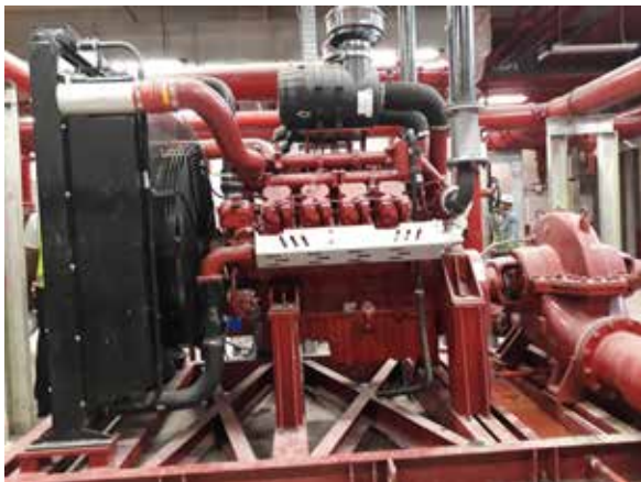
Installation of DV 8 engine for Fire Pump set Application
